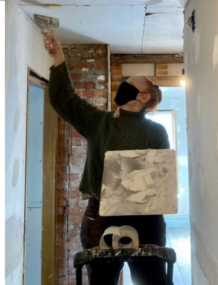
Sandy mudding sheetrock in her house after work.
