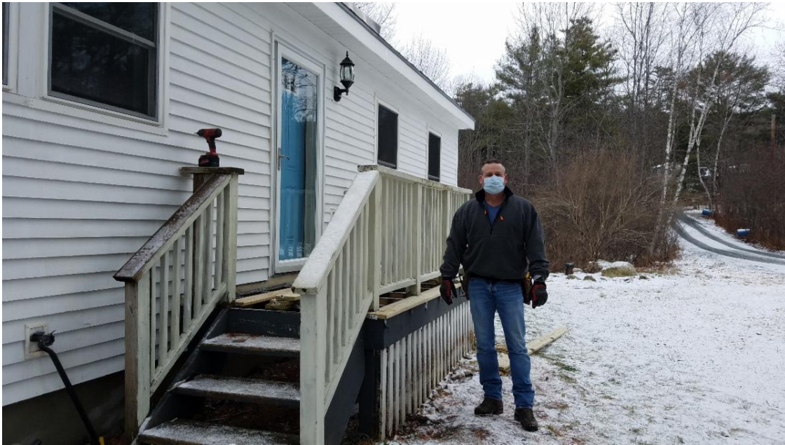
Roger Young Jr. of Hypertherm repairing decking in early December.
