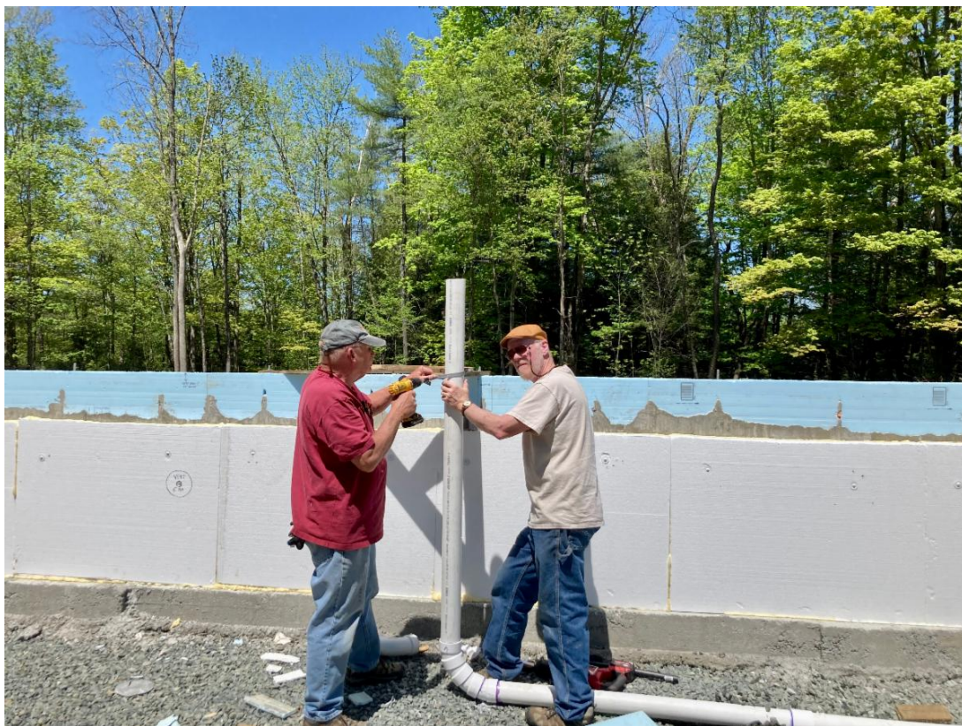
Dave Sherman & Todd Lloyd work together on plumbing rough-in
