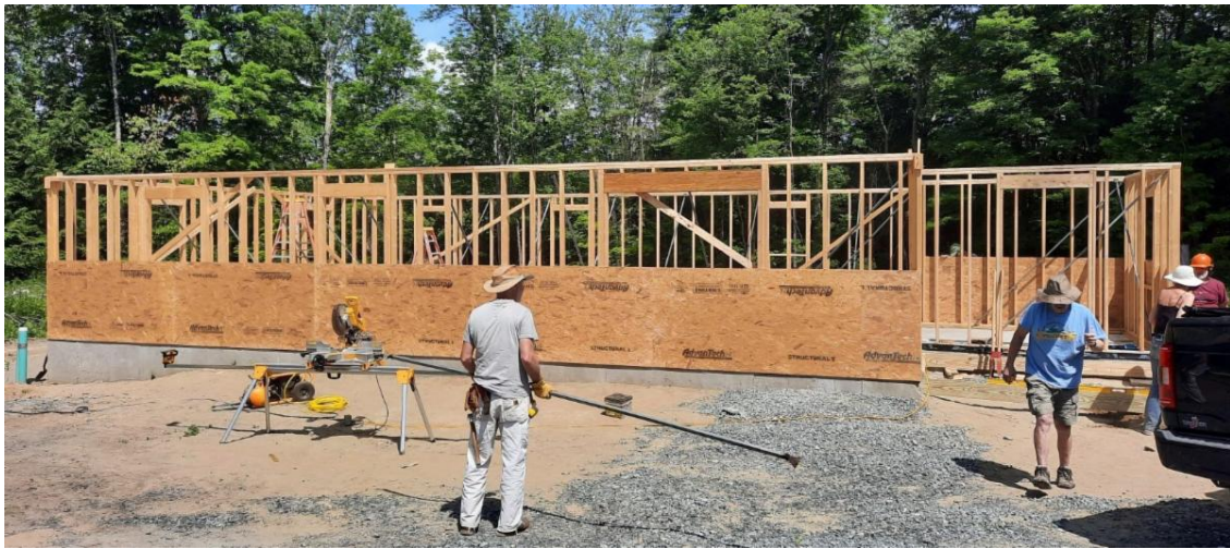
A group from St. Thomas Church and "regular" volunteers frame, sheath, and prep for the deck.
