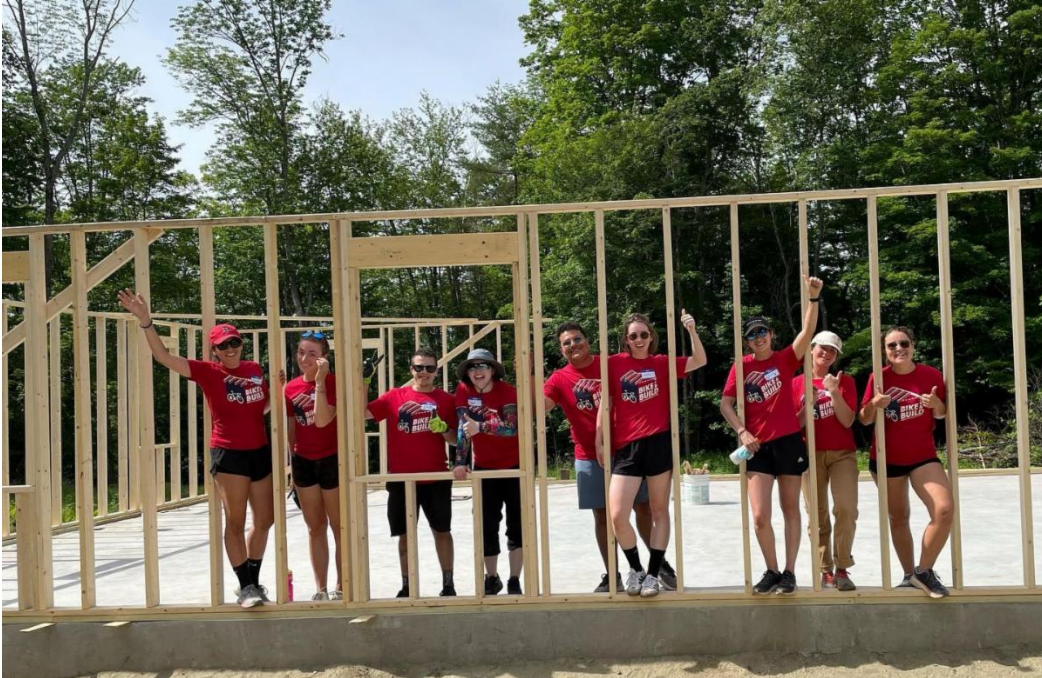
The Bike & Build Crew on Site in mid-June
