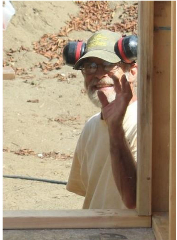
Jim on the construction site in Sharon, VT in 2018
