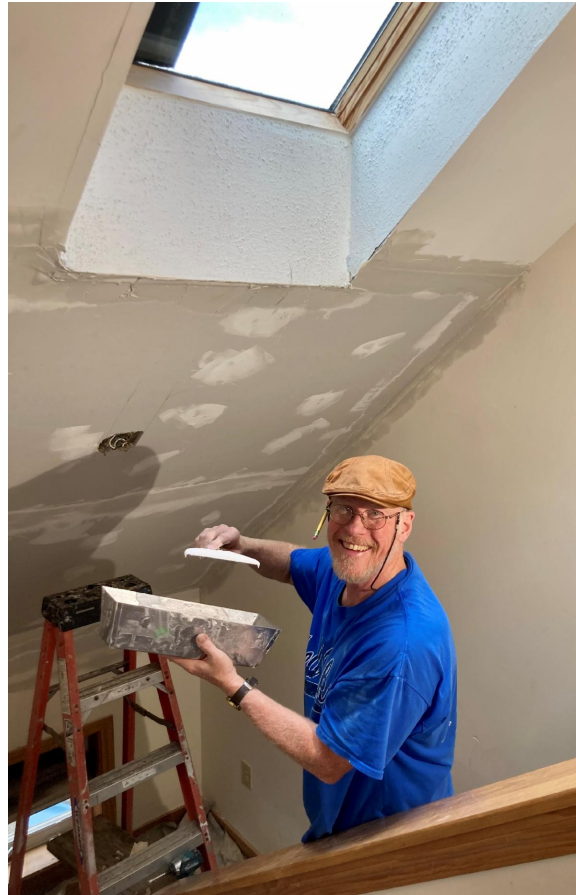
Todd taping Sheetrock at Susan's house.
