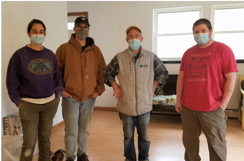
Adriana Lucas (board member); Sean Columbia (Hypertherm); Jim Masland (Site Supervisor) & Rick Rheume (Hypertherm) take a lunch break from interior renovations at the Chin Family home in Lebanon.
